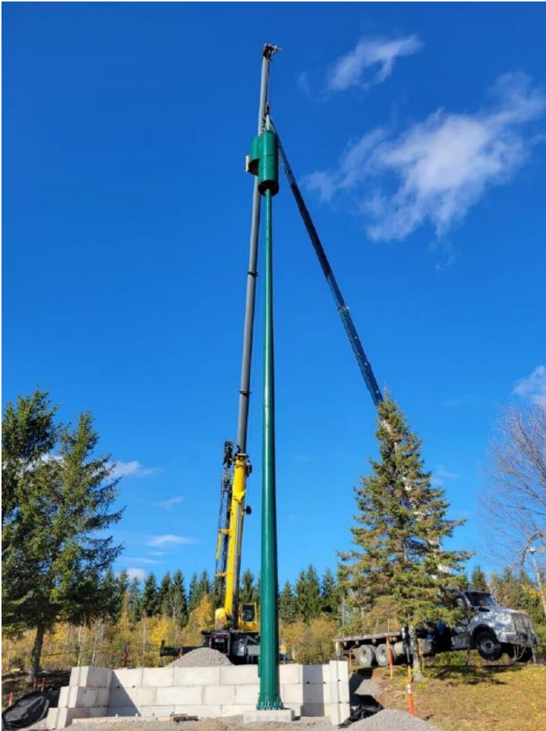
Figure 1: Installation of a tower with similar design
