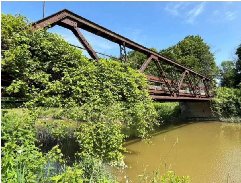
Figure 12: East elevation, looking northwest (A.S.I., 2024)
