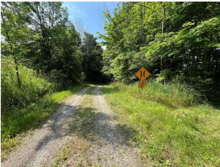
Figure 24: One Lane sign on McKechnie Sideroad north of the subject bridge in a wooded area, looking southeast (A.S.I., 2024)
