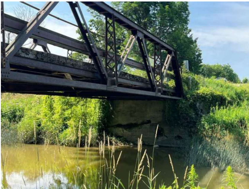
Figure 14: South abutment, looking south (A.S.I., 2024)
