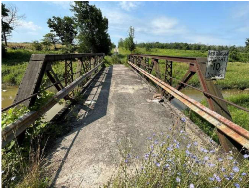
Figure 17: Bridge deck, looking south from the north portal (A.S.I., 2024)
