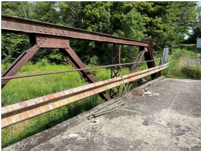
Figure 18: Interior of west truss, looking northwest. Note the flexbeam guardrail and pipe railing (A.S.I., 2024)
