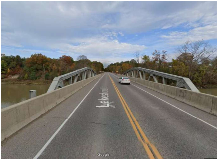
Figure 28: Ausable River Bridge (Google Streetview)
