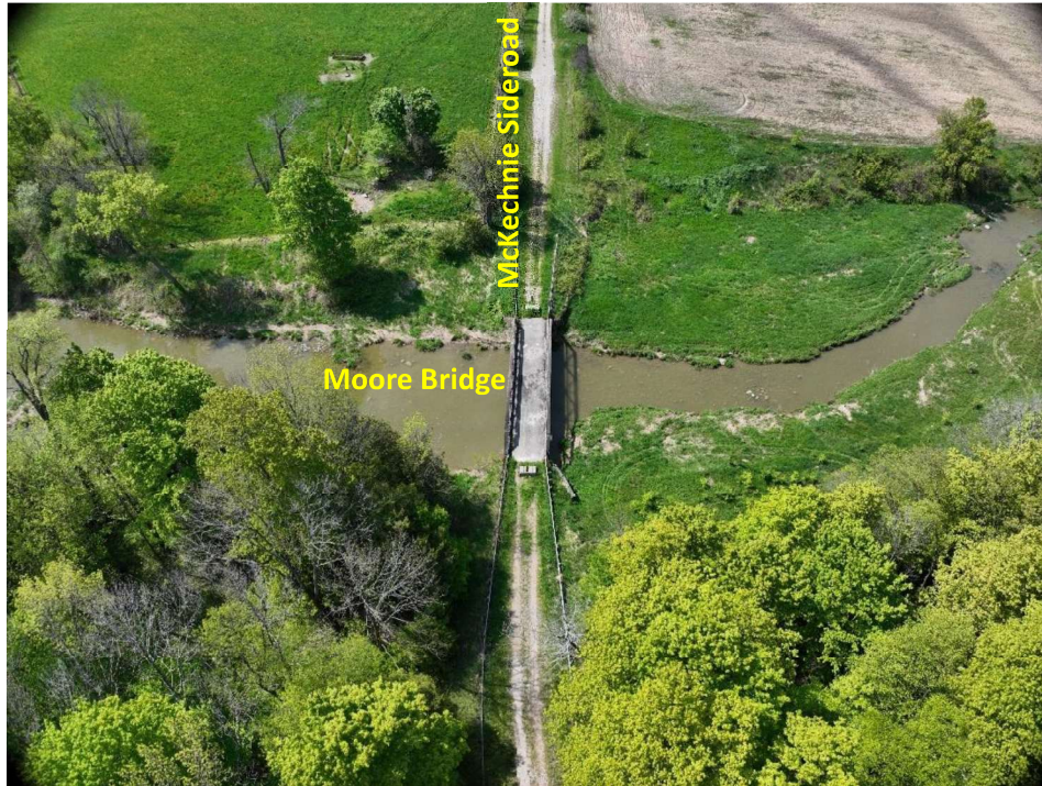
Photo 1: Photo of Moore Bridge showing the single lane road approaches
