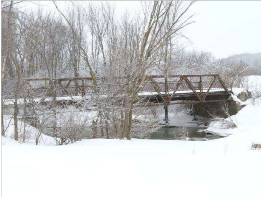
Figure 27: Snake Creek Private Drive Bridge (Holth, 2024b)
