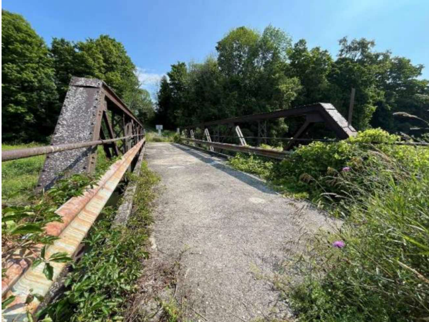
Figure 16: Bridge deck, looking north from the south portal (A.S.I., 2024)
