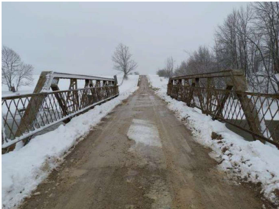
Figure 29: B Line Bridge over Snake Creek (Holth, 2024a)
