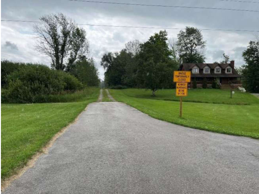
Figure 26: Bridge closure sign at the intersection with Concession Road 8 East, looking south down McKechnie Sideroad towards the subject bridge (A.S.I., 2024)
