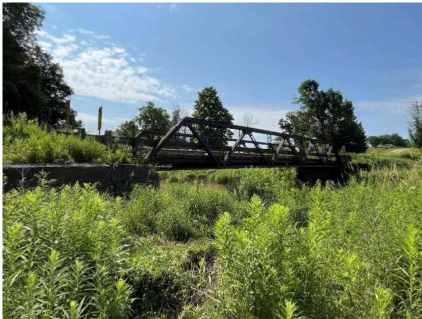
Figure 10: West elevation of Moore Bridge, looking southeast (A.S.I., 2024)
