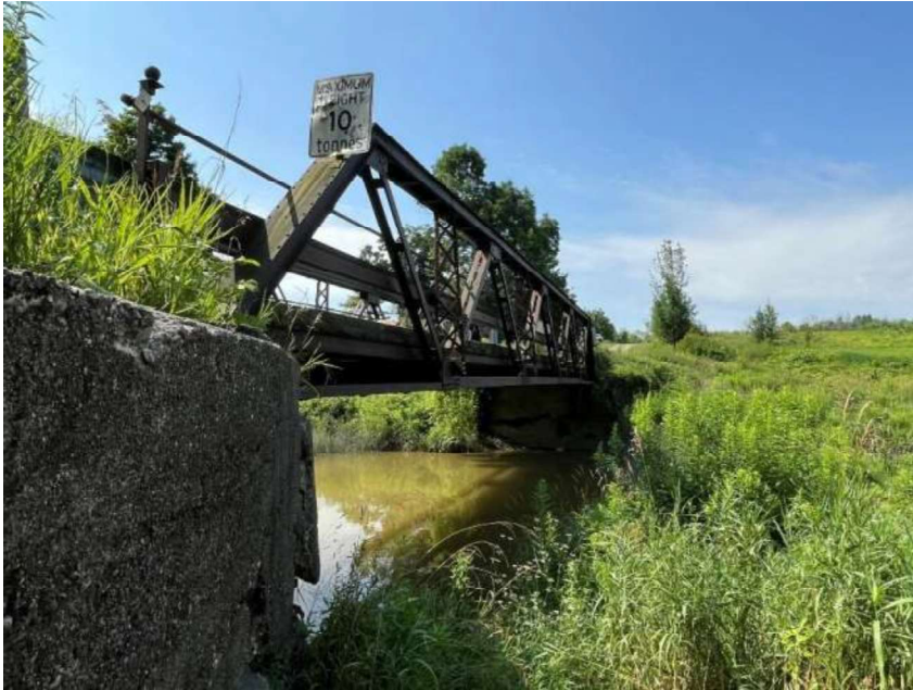
Figure 11: Oblique view of the west elevation, looking south (A.S.I., 2024)
