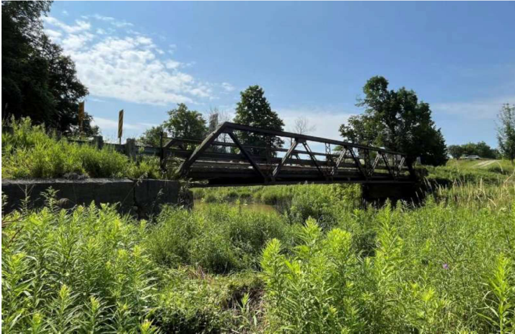
Figure 2: West elevation of Moore Bridge, looking southeast (A.S.I., 2024)
