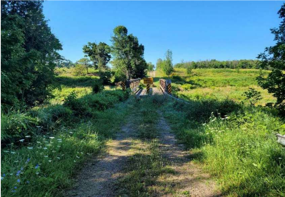
FIGURE 1: OVERVIEW OF STUDY AREA, FACING SOUTHWEST
