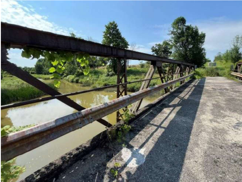
Figure 19: Interior of east truss, looking southeast (A.S.I., 2024)
