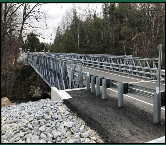
\*Example photos provided by ACROW of a prefabricated steel panel bridge with a steel deck and an asphalt wearing surface.
