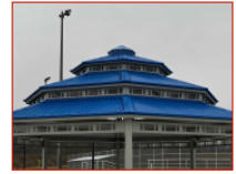
STANDING SEAM METAL ROOF COLOUR TO MATCH THAT OF THE EXISTING SHED
