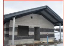
TWO-COLOUR CONCRETE BLOCK WALL WITH METAL ROOF FRAMING
